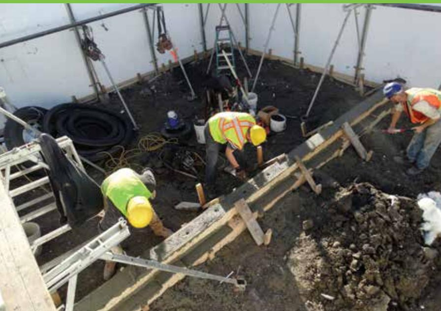
Workers constructing RRC experimental house being divided in two equal sections. The house tested the properties of TDA compared to natural material behind foundation wall and under concrete slab floor.
