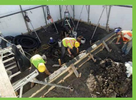
Workers constructing RRC experimental house being divided in two equal sections. The house tested the properties of TDA compared to natural material behind foundation wall and under concrete slab floor.
