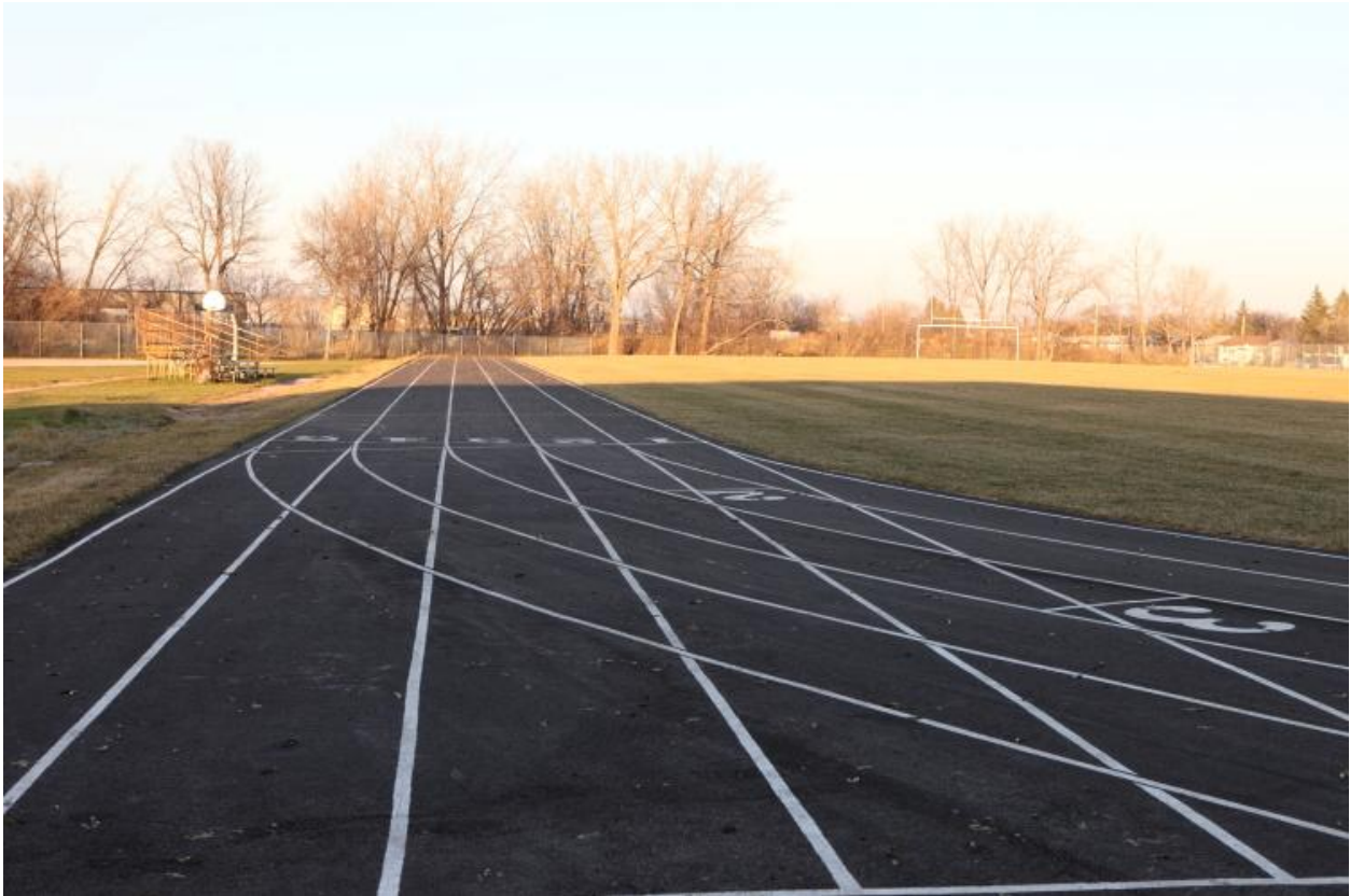
Rubber Asphalt Athletic Track, Elmwood High School, Winnipeg
