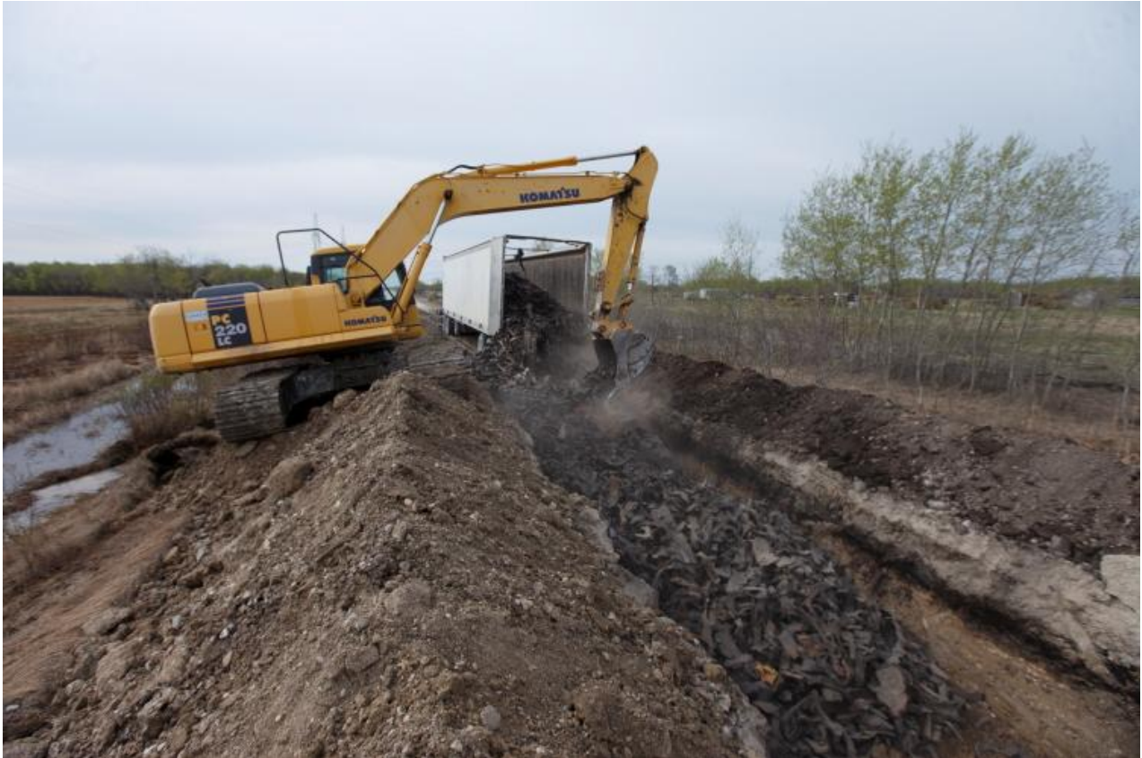
Scrap Tire Derived Aggregate for municipal road remediation – OTR Recycling, Ashern
