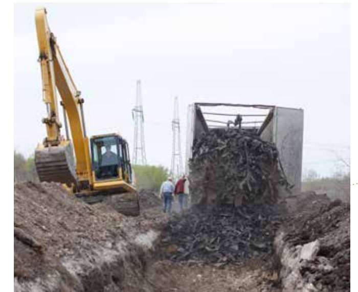
Installing TDA at Silver Bay Road, RM of Siglunes
