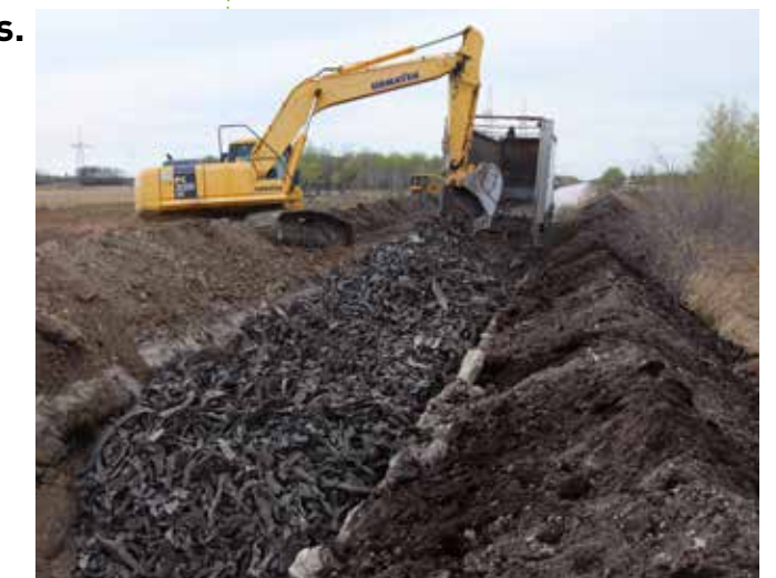
Installing TDA at Silver Bay Road, RM of Siglunes
